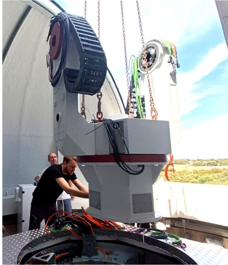
Telescope assembly installation: cable wrap, mount and telescope receiver (from left to right)
